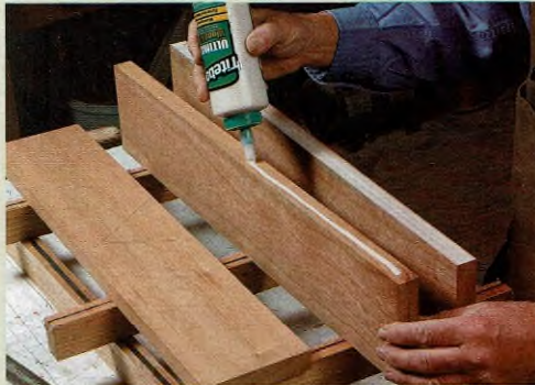
Apply glue straight from the bottle when possible. If the joints are freshly cut, you only have to apply glue to one of the mating surfaces in each joint.
